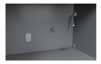
4. Route the power cables and hoses through service holes. Ensure power will remain accessible following install to allow access for any future product maintenance.
