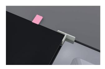
**2.** Place the shims on top of the product to gauge what thickness is required to create a level installation.
