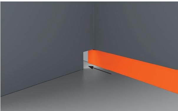
2. If possible, cut a piece of foam to line the back wall adjacent to the dishwasher.
