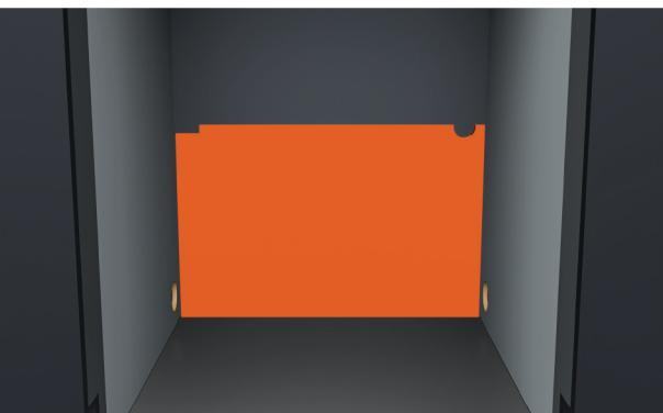
4. Peel half of the backing off at the bottom of the foam. Start at the bottom where the wall meets the floor and continue to peel the backing off as you move upwards.
