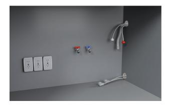
11. Route the power cables and hoses through service holes. Ensure power will remain accessible following install to allow access for any future product maintenance.
