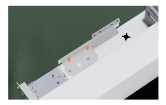
**5.** For the non-hinge side, fit a new alcove bracket using M6x16 countersunk screws.
