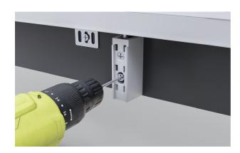
2. Slot flow divider onto the screw at the base of the door. Secure using the supplied screws.
